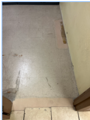
Encapsulation of Asbestos
